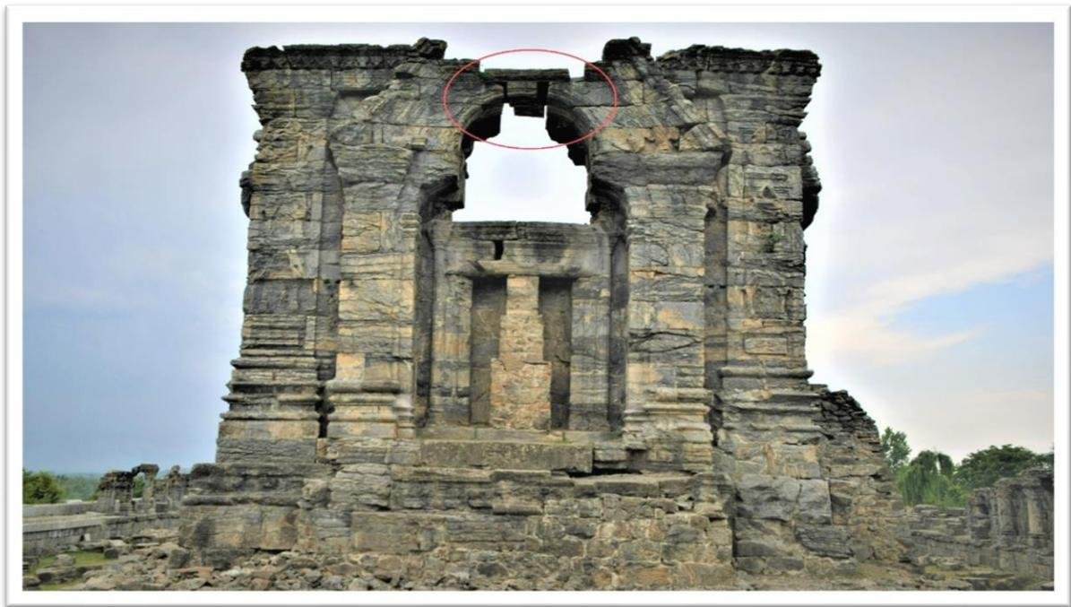
**Fig. 3: Rear View of Sun Temple, Martand, with evidence of true Arch**
